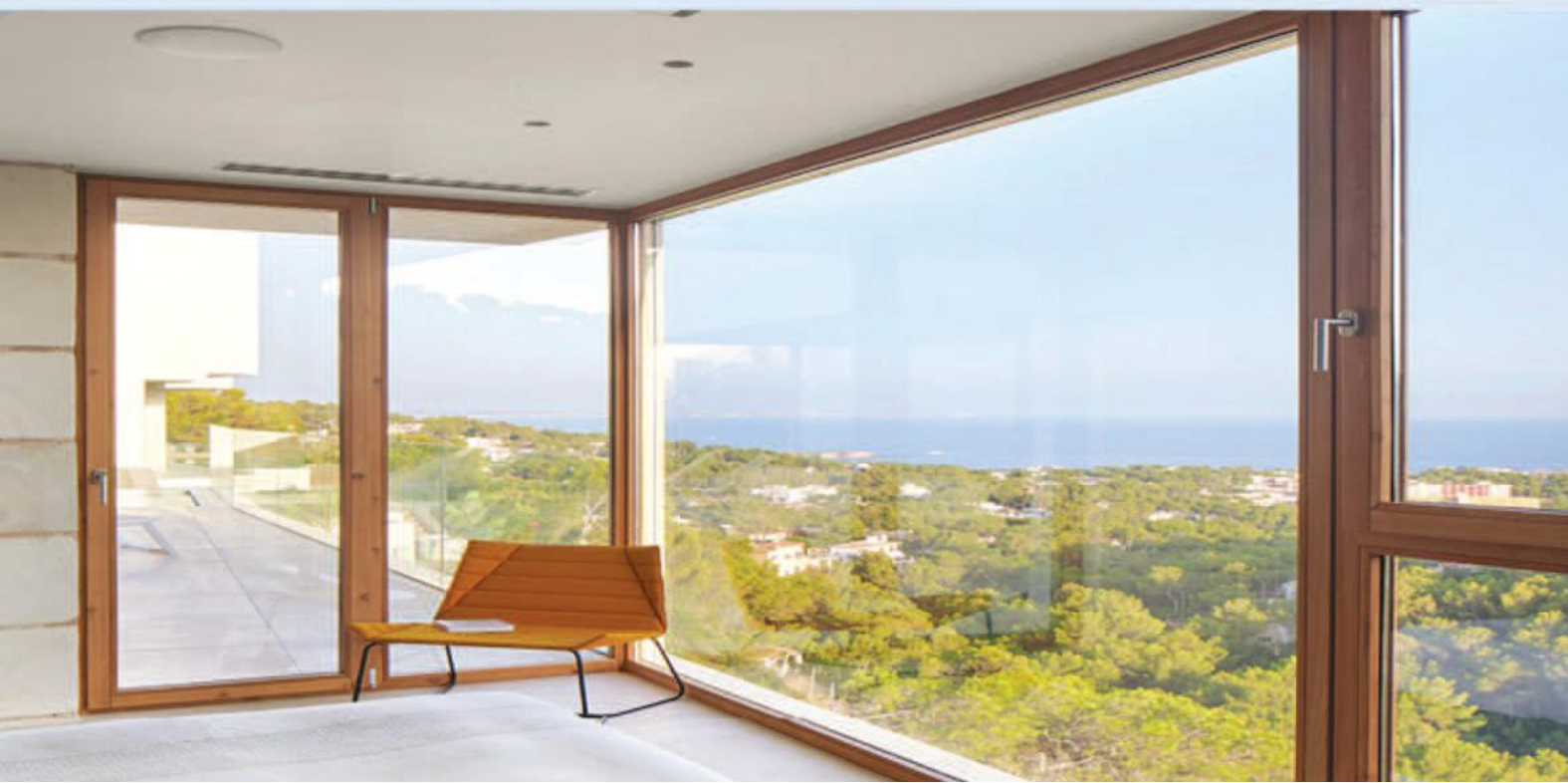
WOODEN WINDOW WITH EXTERIOR ALUMINUM CLADDING
